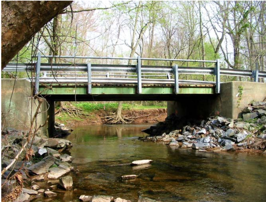
Existing White Ground Road Bridge
