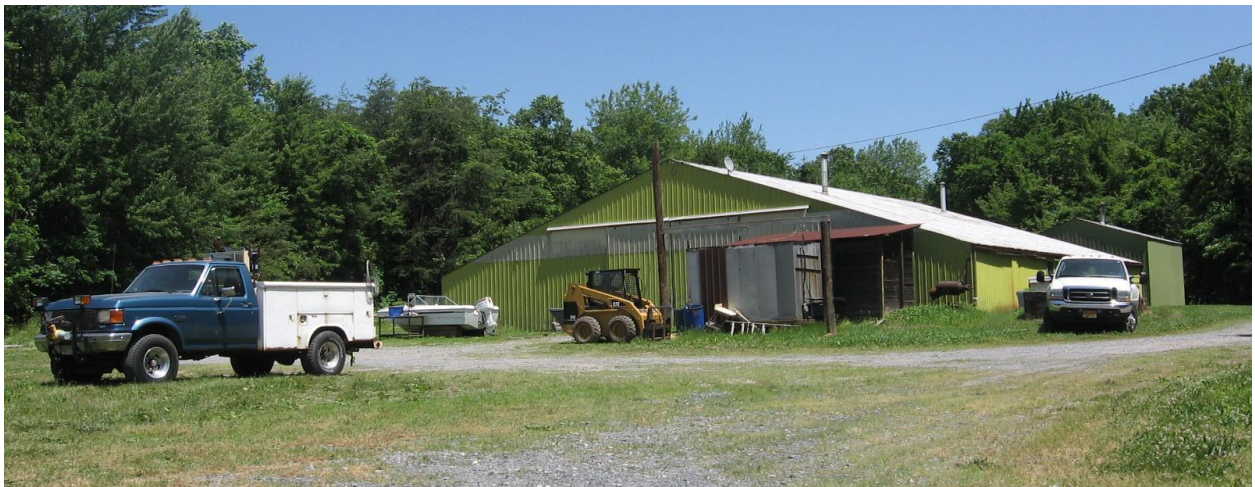
Buildings currently on property (three photos)
