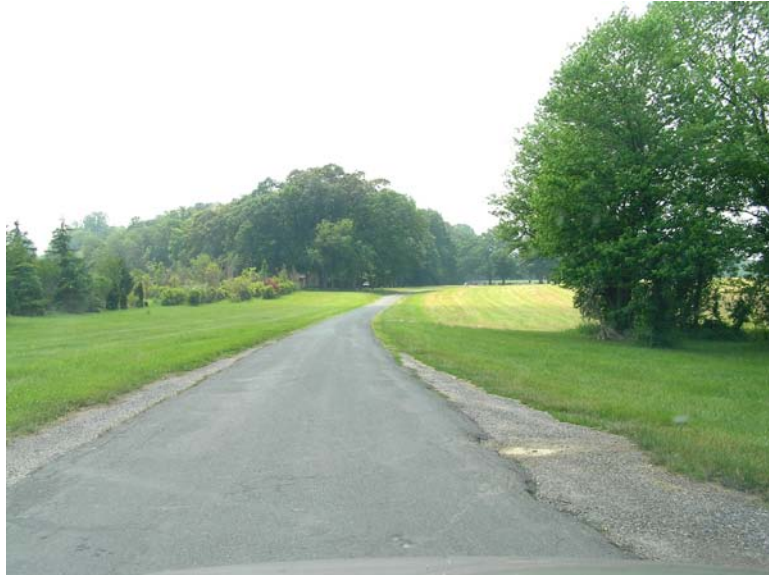
Mt Carmel Cemetery Road appears to meet the requirements for a rustic or exceptional rustic road designation.
