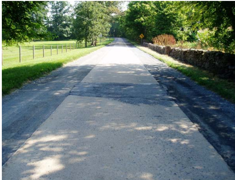
Martinsburg Road, a politicians road and the only road designated in the Master Plan for Historic Preservation, shows extensive damage and patching.
