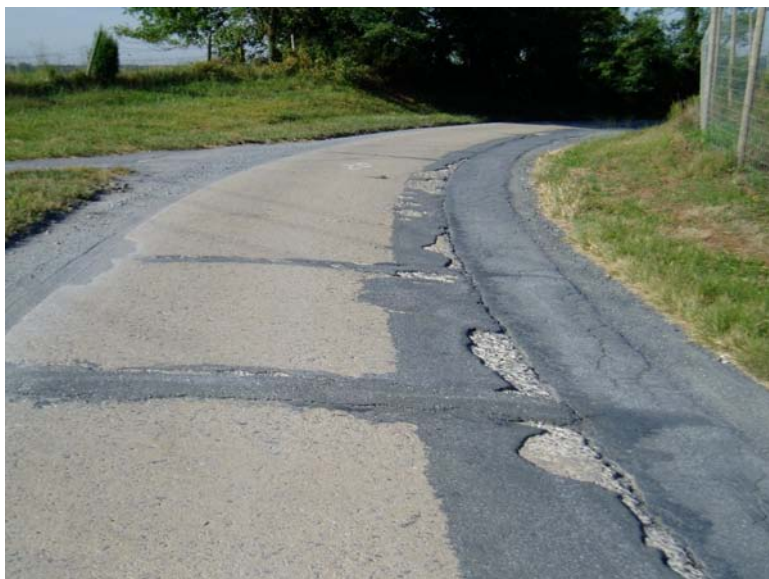
Sugarland Road, also a politicians road, has been damaged and patched much like Martinsburg Road
