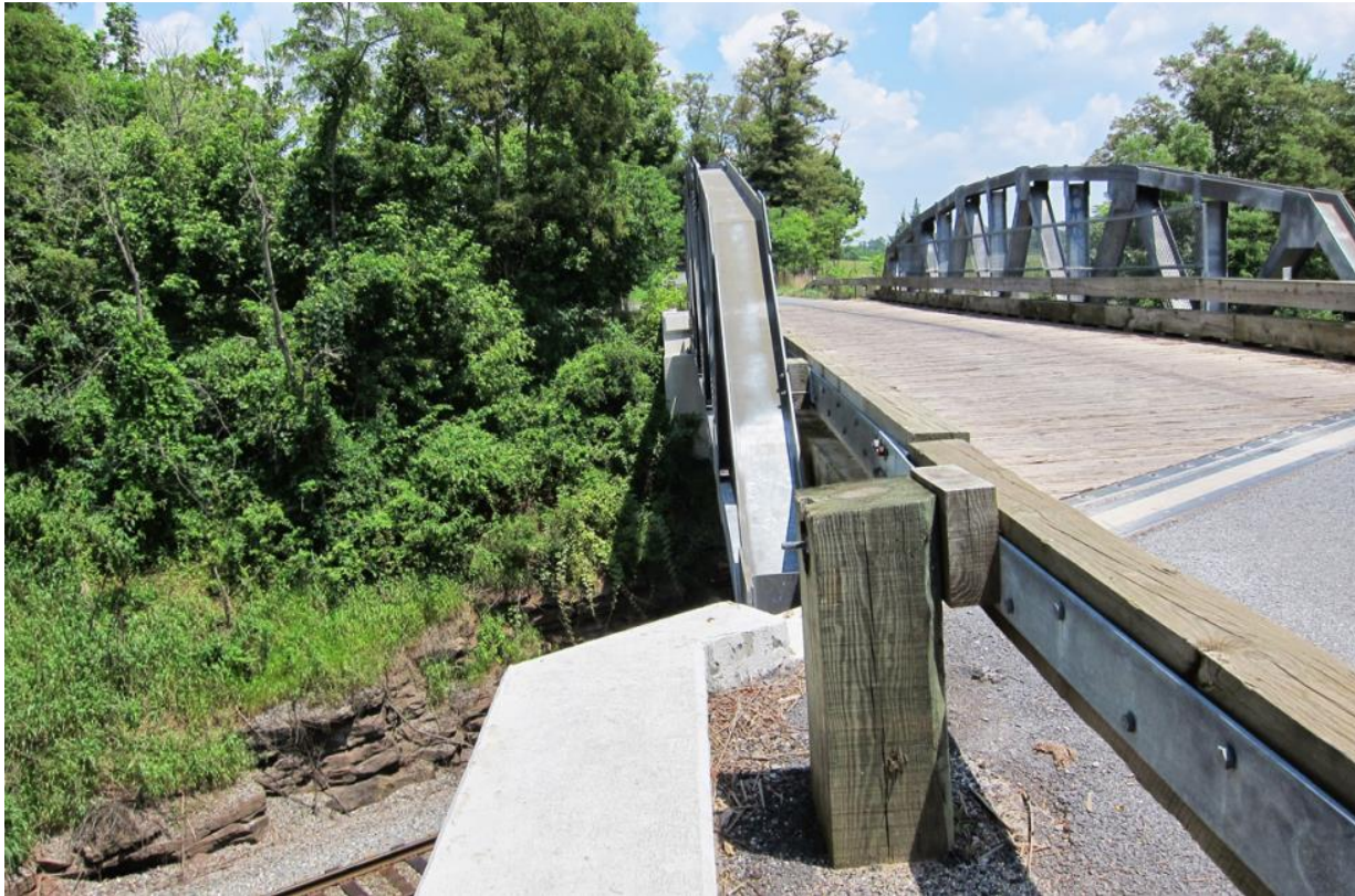
Steel-backed timber guardrail used on the Mouth of Monocacy Bridge.
