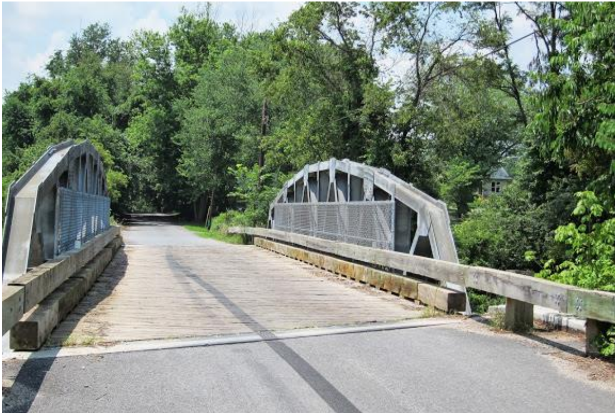
This replacement bridge at Mouth of Monocacy Road over the CSX railroad follows the profile of a pony truss, and is sympathetic to its rustic surroundings.
