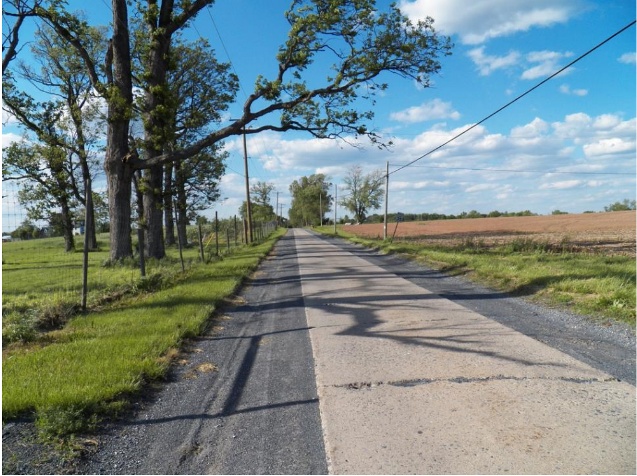
Proper maintenance of the historic concrete sections of the politicians' road along Sugarland Road has helped protect this 1930s era pavement.
