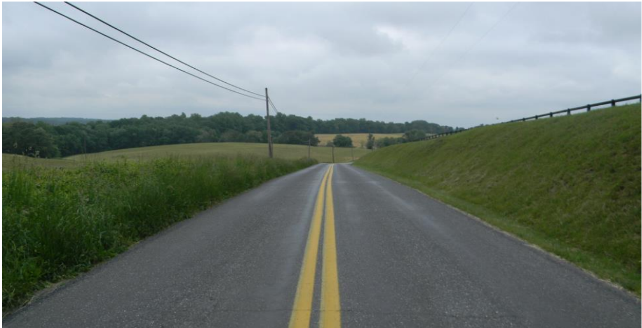
Comus Road is an example of a Rustic Road with “outstanding agricultural and rural vistas,” as they are described in the RRFMP.
