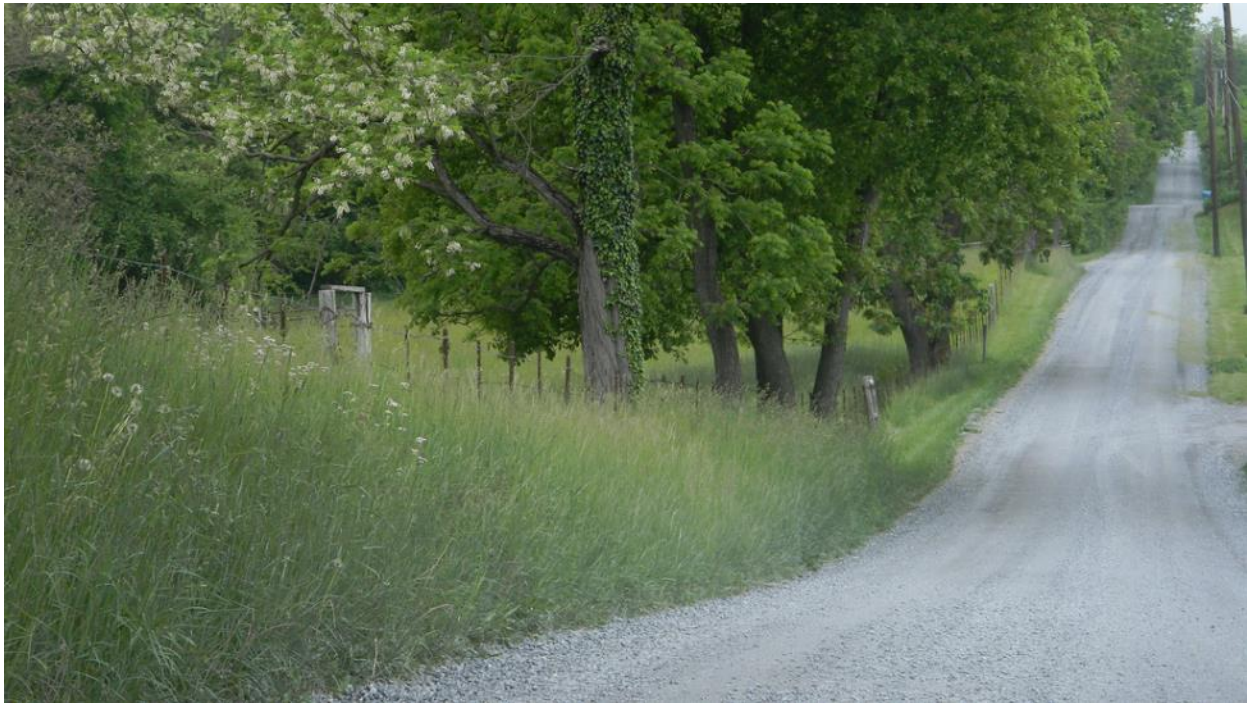
The gravel surface on West Harris Road near the town of Barnesville maintains the character of this historic farm wagon road.
