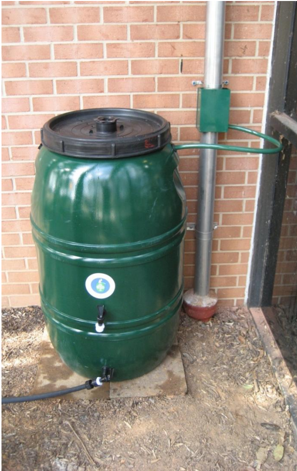
Rockville Senior Center Rain Barrel, Source: Biohabitats
