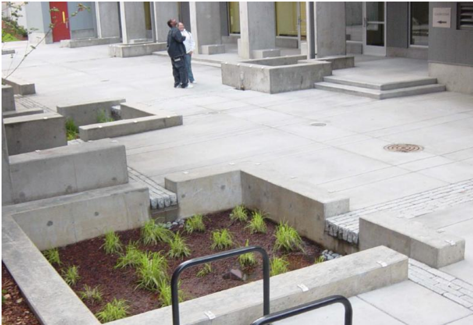
Source: Portland 2004 Bureau of Environmental Services Manual, Appendix H: Stormwater Management Facility Photos, September 2004 Stormwater Management. http://www.portlandonline.com/BES/index.cfm?c=35122 Manual.
