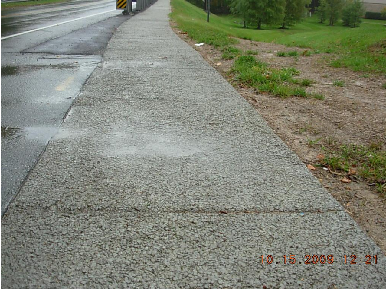
Good Hope Road pervious concrete sidewalk, DOT
