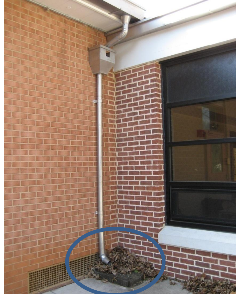
Gaithersburg Community Center, Source: Biohabitats
