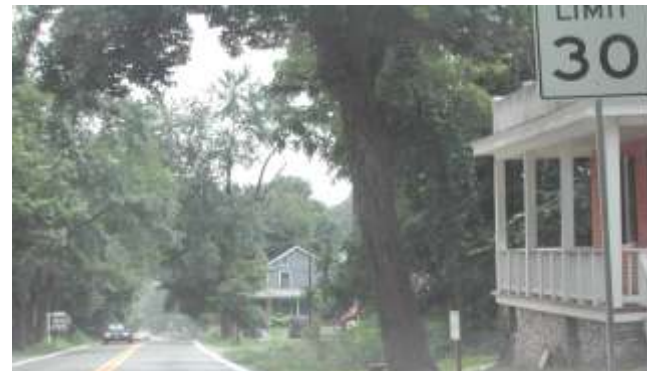
Two Lane MD 355 rural road, Hyattstown
