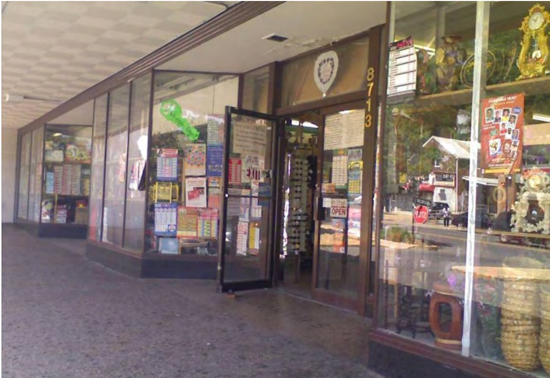
The Woolworth storefront (8713) has a high level of integrity with original window walls, black marble base, and ribbed metal cornice. Terrazzo Floor (below). (Clare Lise Kelly, M-NCPPC, 6-2010)
