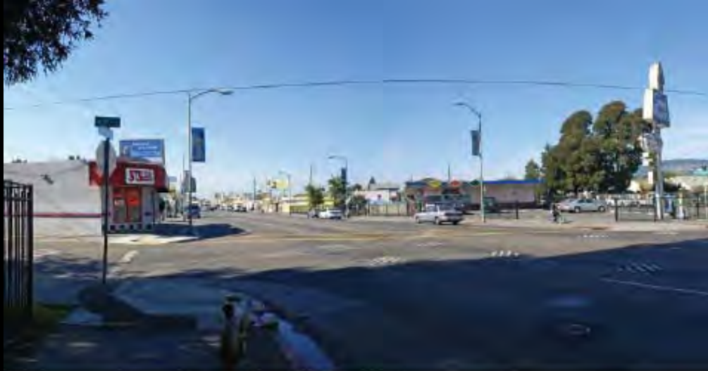
Existing condition of International Blvd at 81st Ave.
