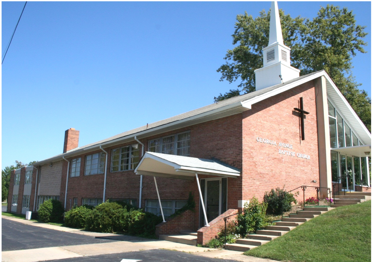
FIGURE 7 - West corner of building. Northwest side (left) faces Glenallen Avenue. Clare Lise Kelly, September 12, 2012
