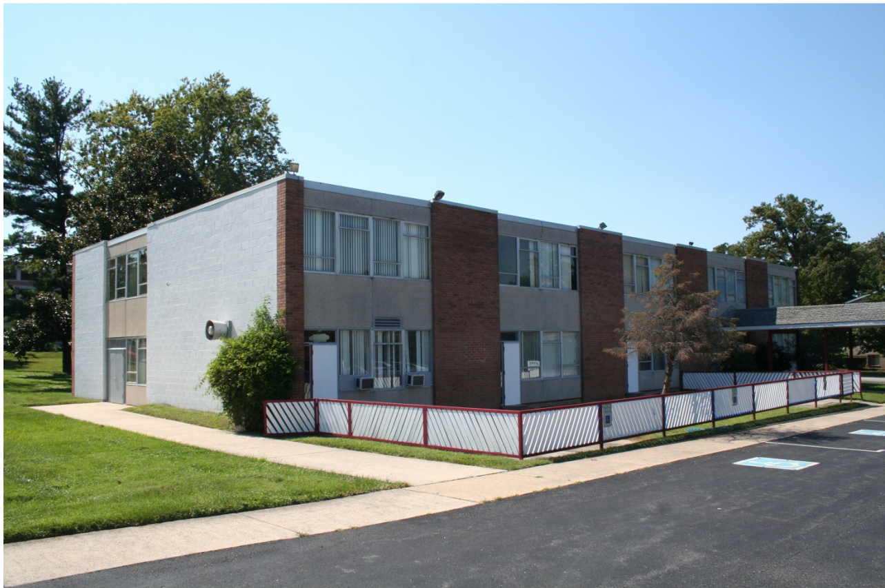
FIGURE 11 - East corner of education wing. The fence, with steel frame and diagonal wood slats, is original, though the wood has been replaced. Clare Lise Kelly, September 12, 2012
