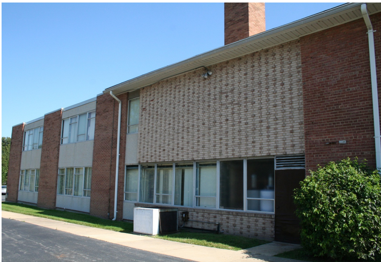
FIGURE 8 - Northwest façade: Auditorium block extension (center) and education wing. Clare Lise Kelly, September 12, 2012
