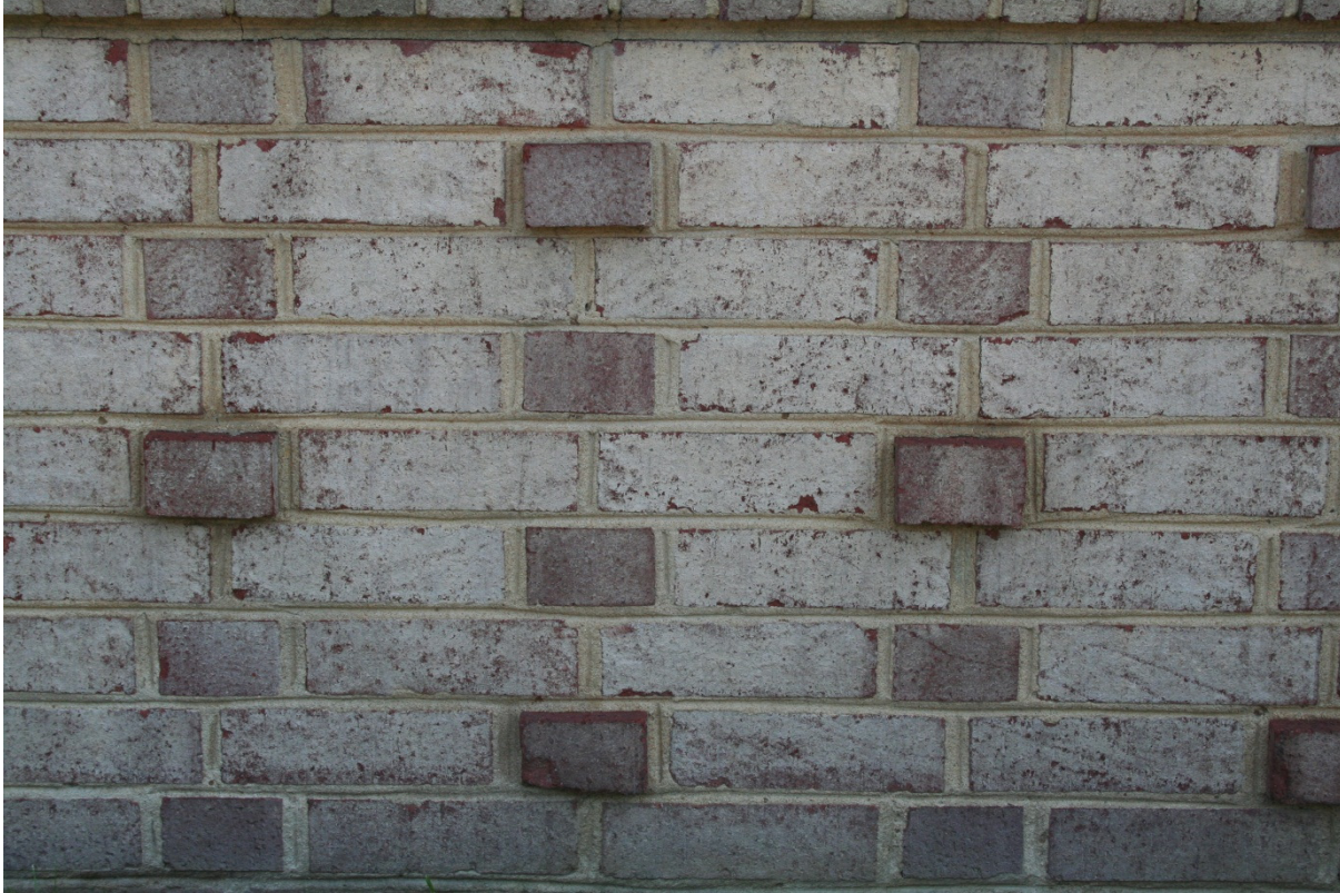
FIGURE 13 - Detail, Brick wall on 1962 Auditorium extension with protruding headers on alternating courses
