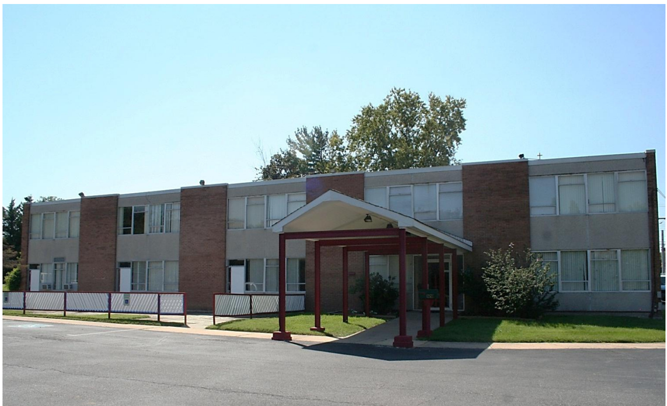
FIGURE 10- Rear (northeast) façade of Education Wing (1962), Clare Lise Kelly, September 12, 2012
