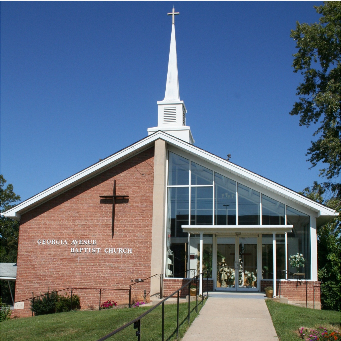
FIGURE 5 - Auditorium (1956), Front (SW) Façade, Clare Lise Kelly, September 12, 2012
