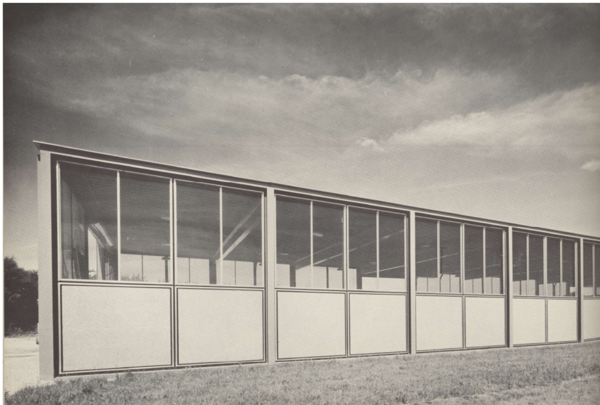
FIGURE 26 - Charles Goodman featured TECFAB panels in his award-winning design of the TECFAB plant in Beltsville. The structure has since been demolished. (Source: The Architecture of Charles Goodman Associates, company brochure)
