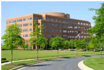
Multi-story office building in the Milestone North Business Park.
