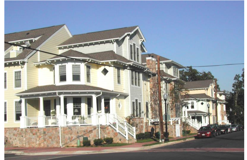
Varied roof lines on residential development, Clarendon, Virginia
