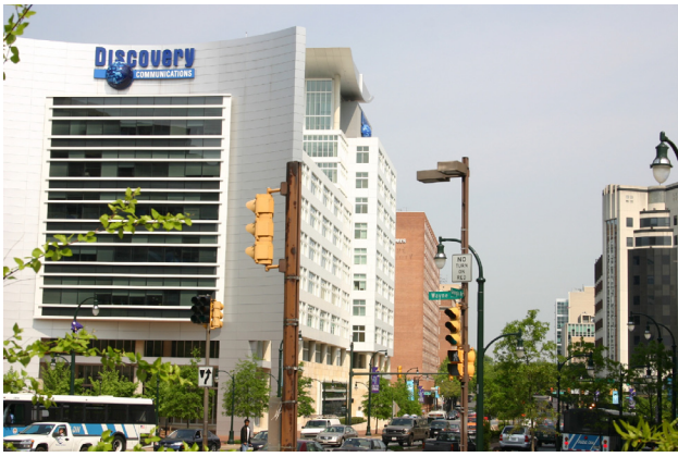
Georgia Avenue looking north at Wayne Avenue.
