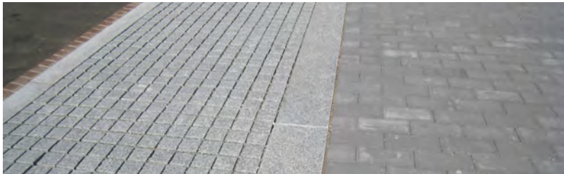
Permeable pavers in seating areas along trail
