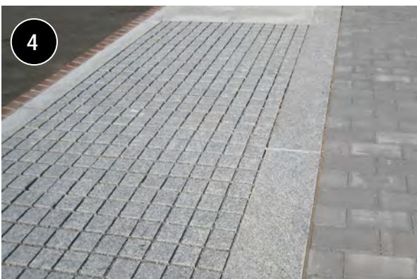
Permeable pavers in seating areas along trail
