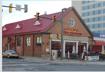
Adaptive Reuse: From a fire station to a restaurant
