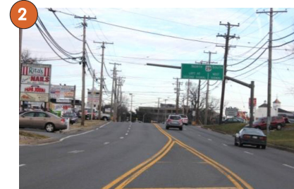
2 Lack of sidewalks
