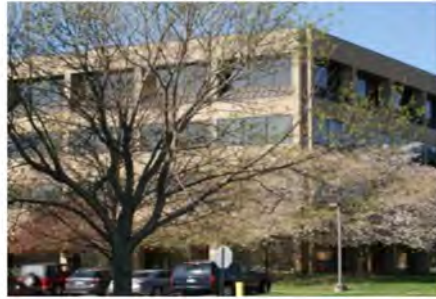
Offices along Business 29
