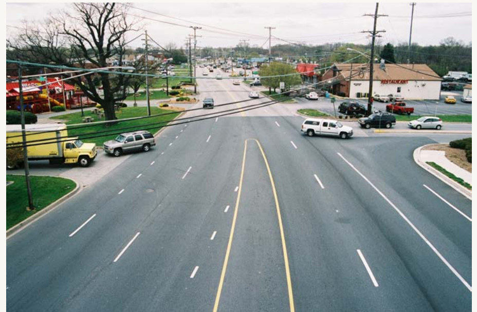
MD 198, looking west Timothy Hyman, Maryland State Highway Administration
